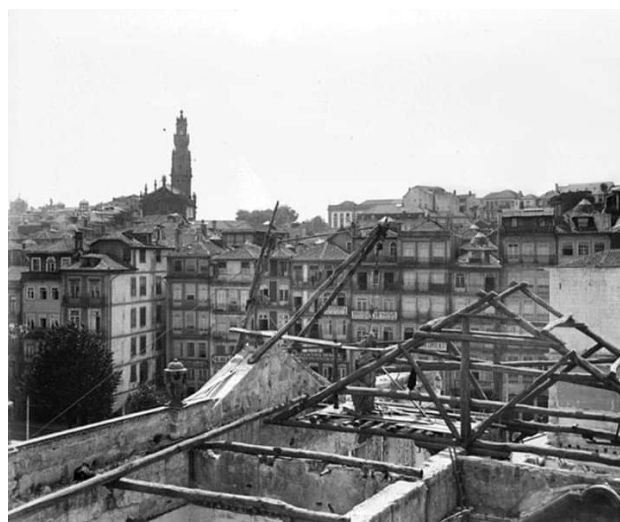
Fig. 17 Photos from the demolition process in 1916
