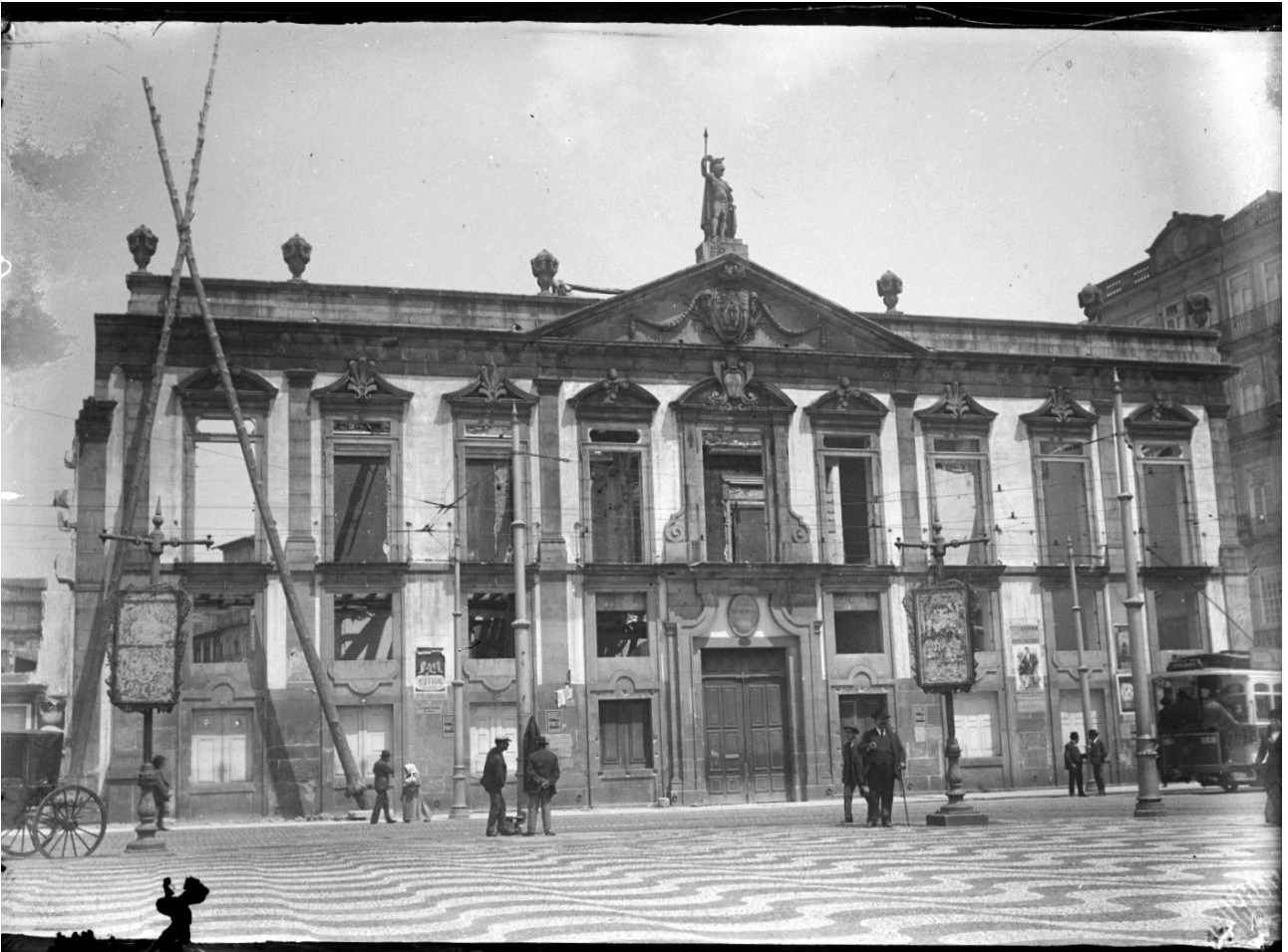
Fig. 21 Photos from the demolition process in 1916
