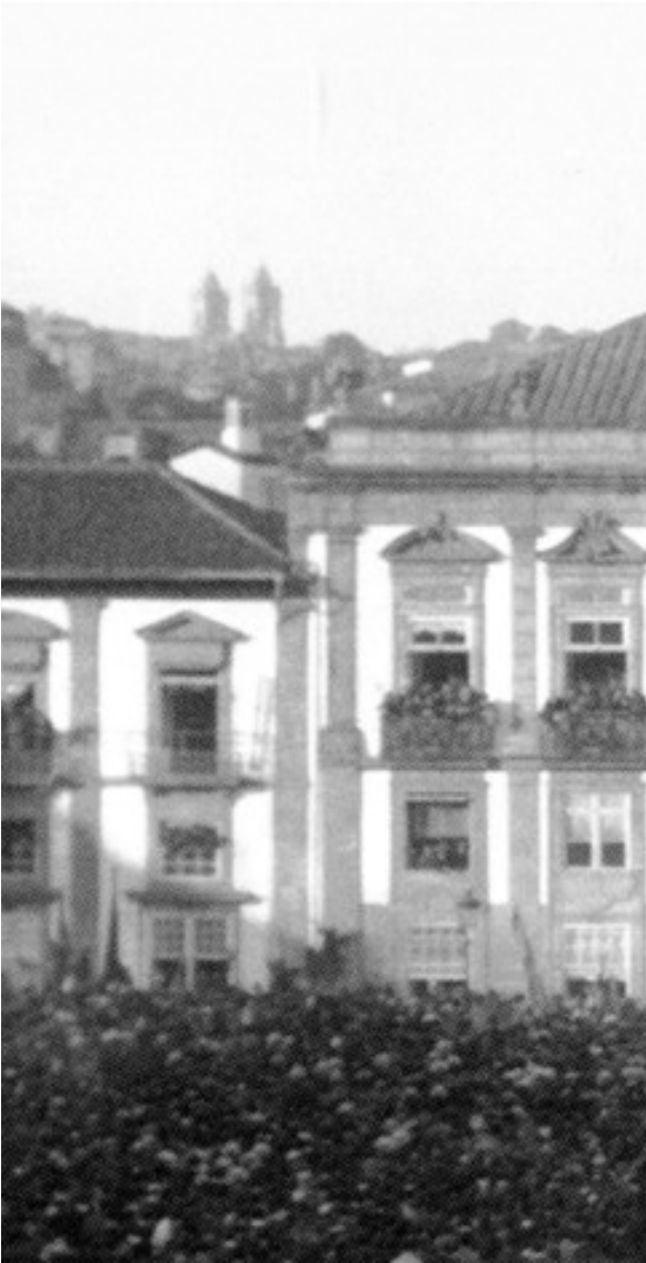
Fig. 12 Southern Elevation detail
