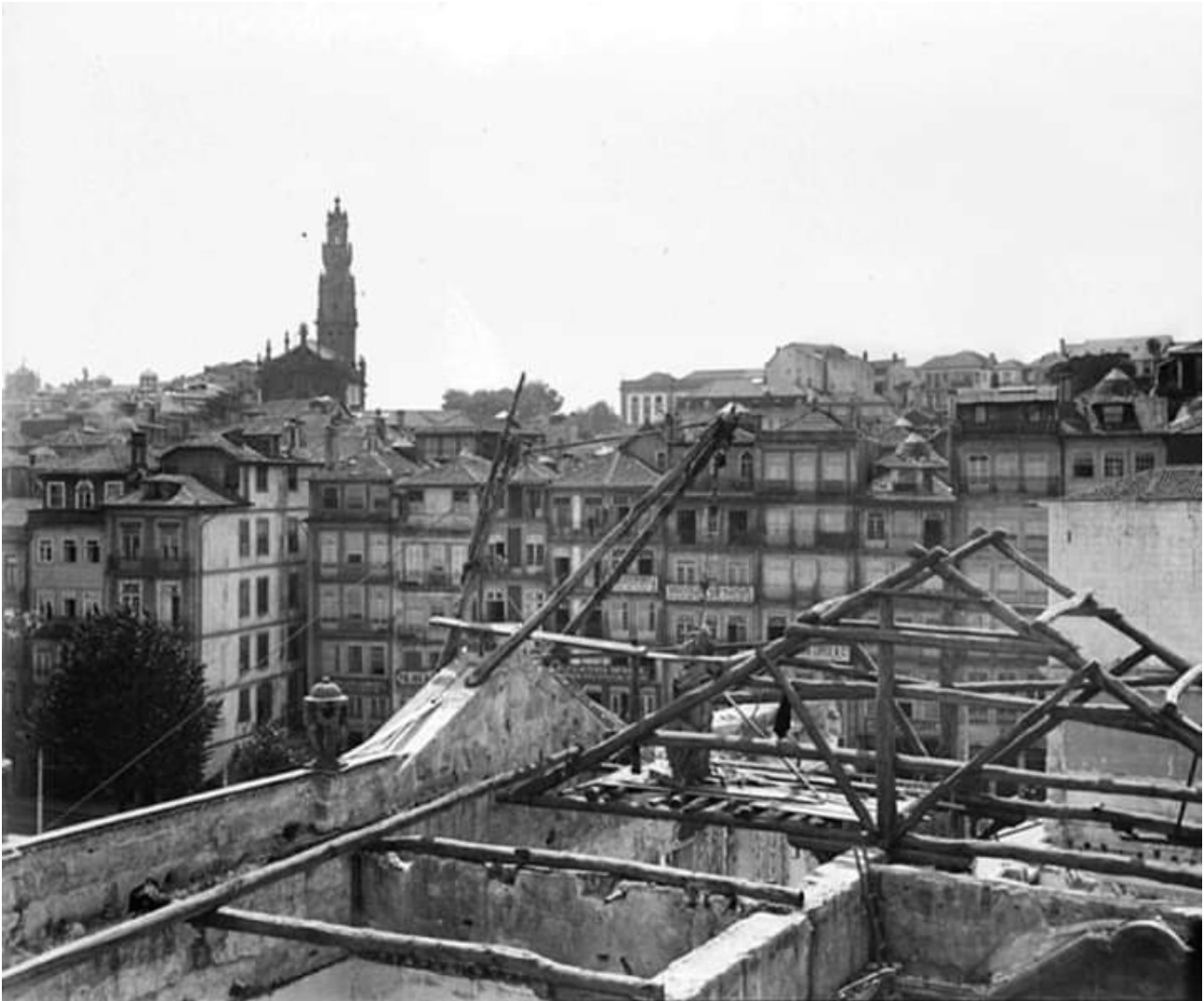
Fig. 17 Photos from the demolition process in 1916
