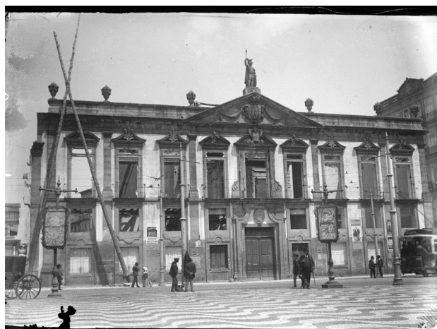
Fig. 21 Photos from the demolition process in 1916
