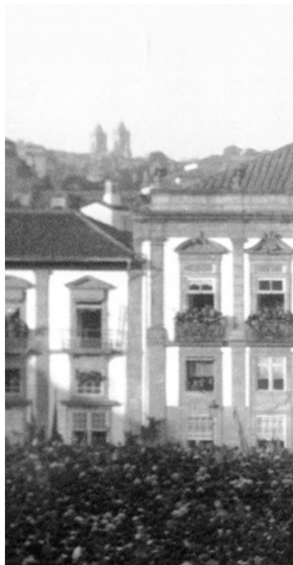
Fig. 12 Southern Elevation detail
