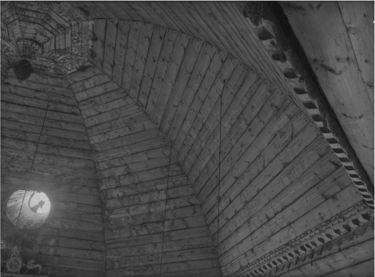
Fig. 15 view of the skylight
