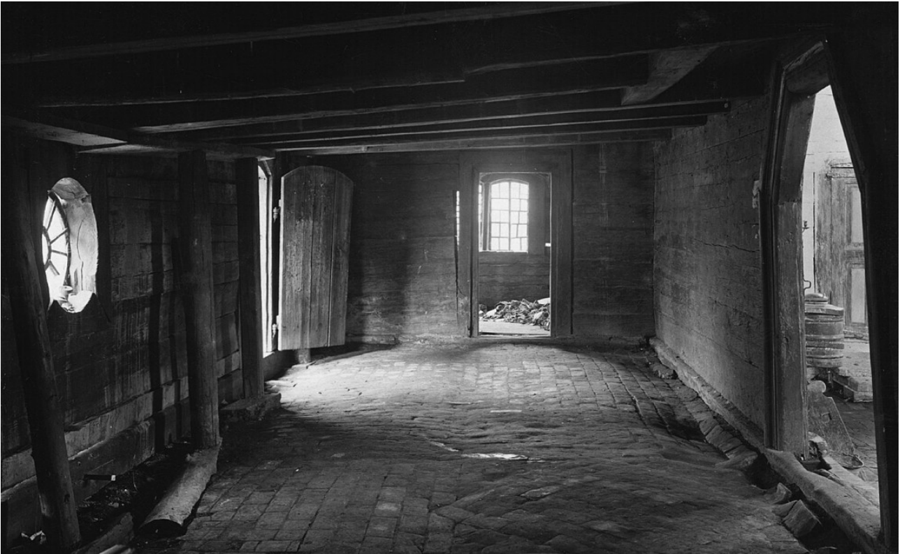
Fig. 12 Interior of the vestibule
