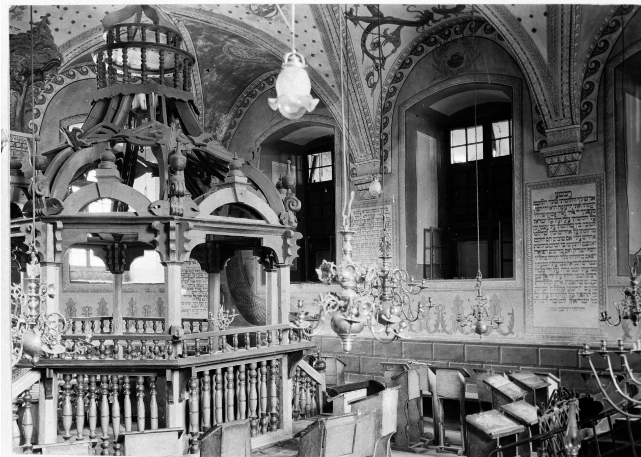
Abb. 8 Interior of the main hall state before 1939
