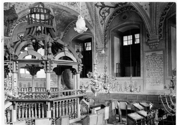
Abb. 8 Interior of the main hall state before 1939
