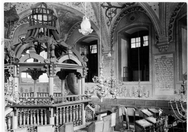
Abb. 8 Interior of the main hall state before 1939
