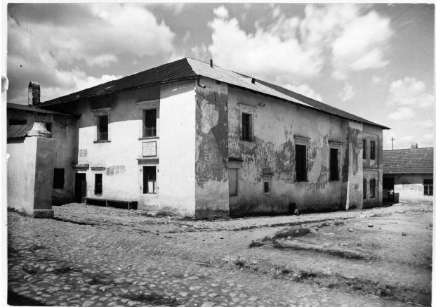
Abb. 6 View from the south-east
