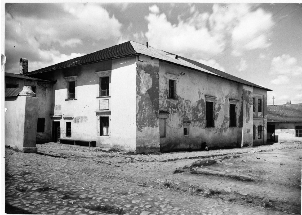
Abb. 6 View from the south-east
