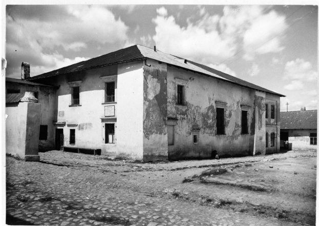
Abb. 6 View from the south-east
