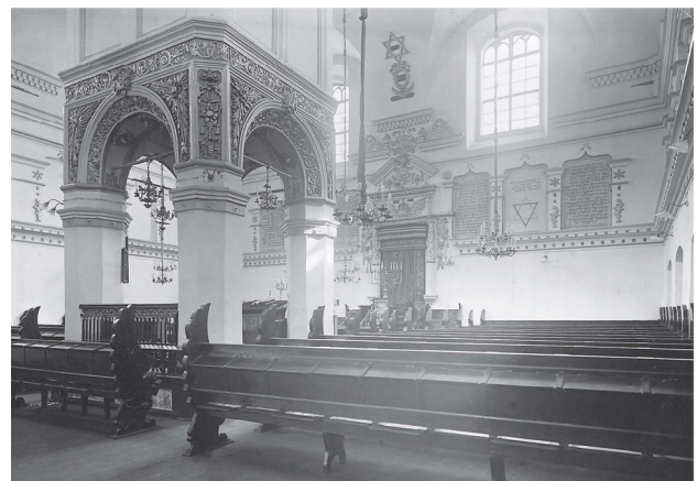
Abb. 32 interior of the main hall, 1925
