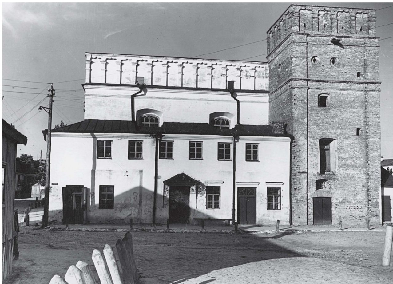
Abb. 31 view from the west, before 1939
