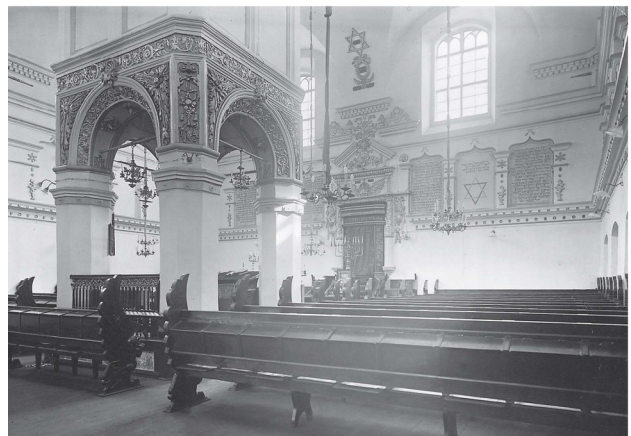
Abb. 32 interior of the main hall, 1925
