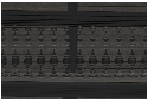
Fig. 42 Balustrades and railings
